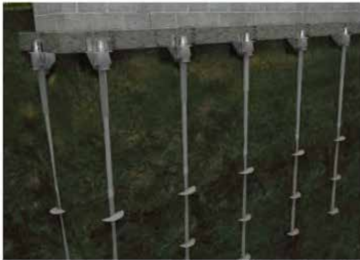
Figure 1.26 Installation of small helical pier
