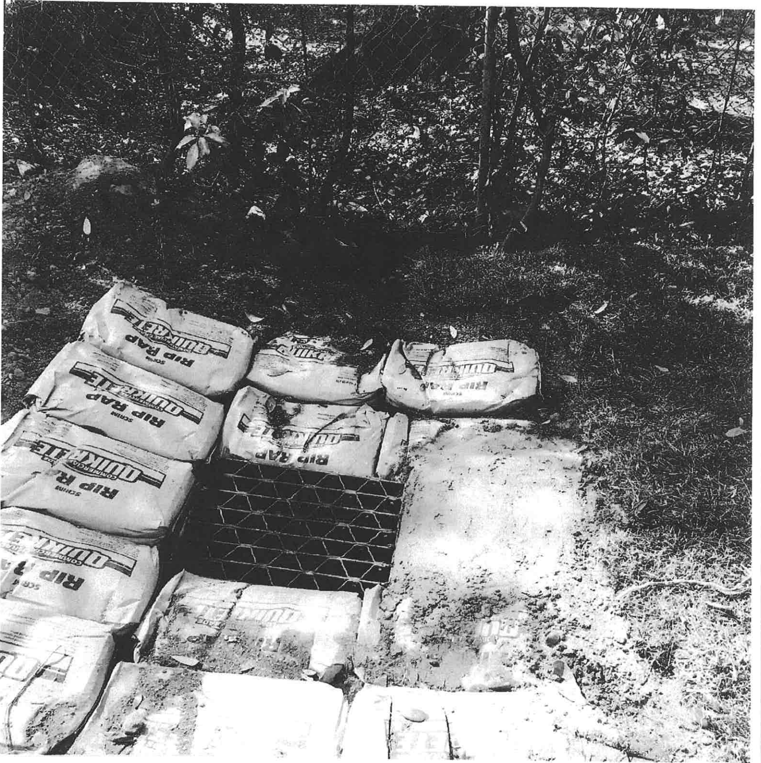
Elm Street After
