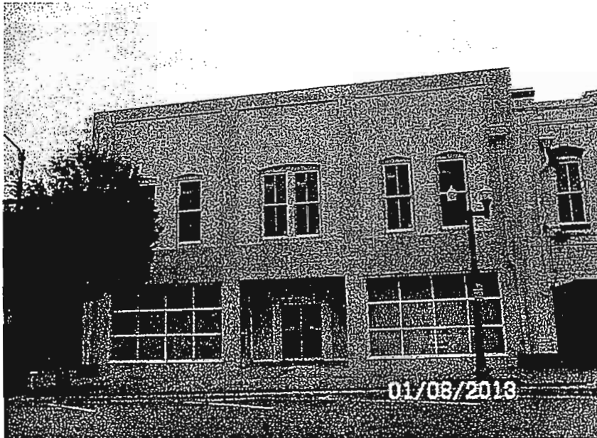
Capital City Bank adjacent building; No. 12 Washington Street
