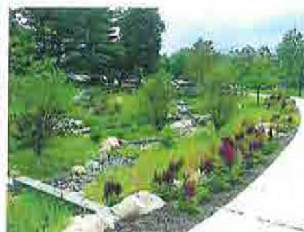
Riparian basin with native plants and stream to slow and filter stormwater runoff
