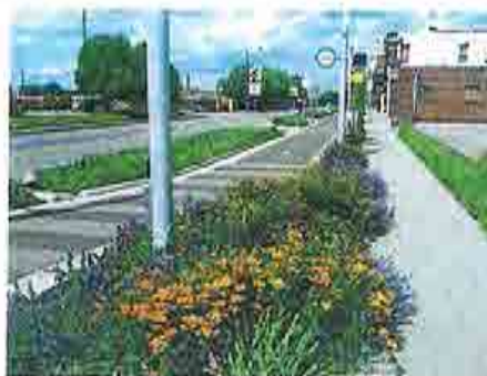
Streetscape with vegetated swales and blue paint and native plantings
